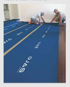
Sheets are designed to provide reusable temporary floor protection for many fixtures and surfaces during construction. The sheets offer excellent surface, tile, vinyl and wooden floors. The sheets are easy to apply and costeffective
